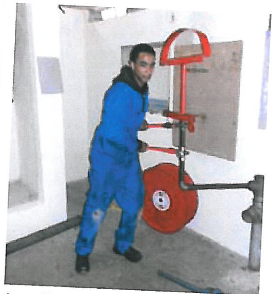
Installing a fire hose reel as part of a practical assessment
