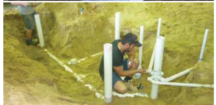
MPA Skills apprentices working in trenches
